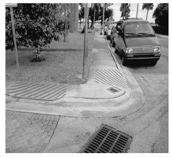
**EXHIBIT V-45**Reducing the curb radius creates a tighter turn and results in motorists making right turns at lower speeds. (Photo by Peter Lagerwey)
