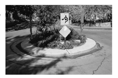
should accompany mini-circles, to discourage motorists from making high-speed right turns. Mini-circles with cuts in splitter islands make crossing easier for pedestrians, especially those in wheelchairs. Larger vehicles, such as fire trucks and school buses, can be accommodated by creating a mountable curb on the outer portion of the circle. Mini-circle landscaping should not block sight distance. Yield controls should be used.
